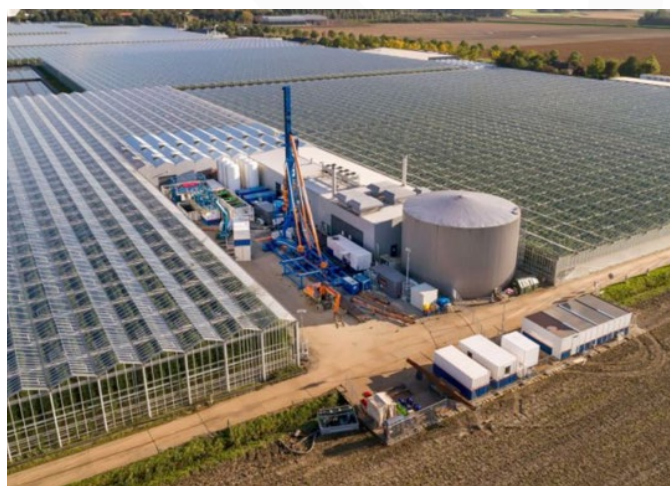
Drilling a Geothermal Well in a Greenhouse Area
